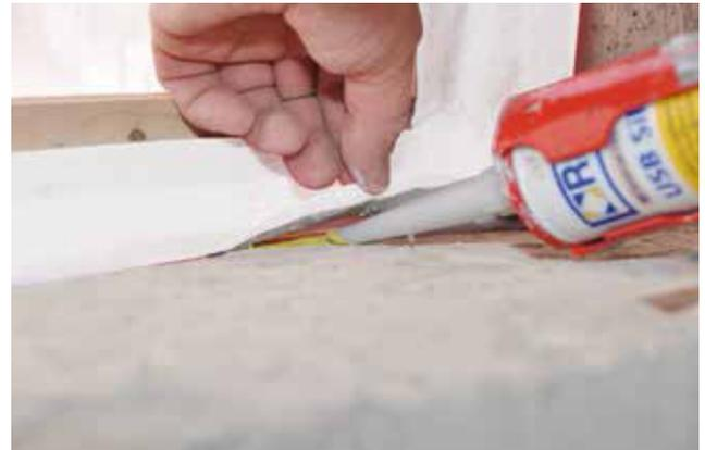
Gluing of external FDB Tape Ext AC tape on masonry
