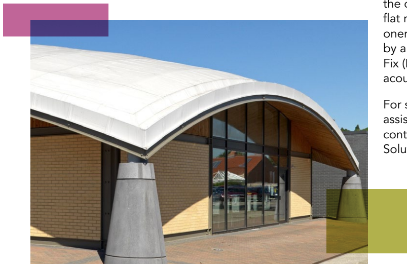
Image courtesy of GSS Architecture - www.gssarchitecture.com
