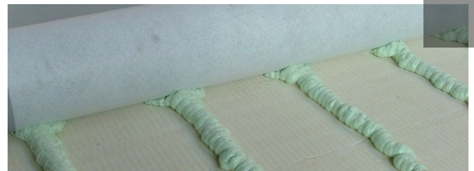
A bonded membrane incorporating HARDROCK® Multi-Fix (DD) Membrane installation/fasteners
