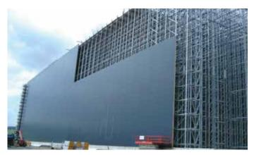
$Fast\ economic\ installation\ of\ the\ Fischer THERM\ sandwich\ elements\ with\ DUO\ sealing.$
