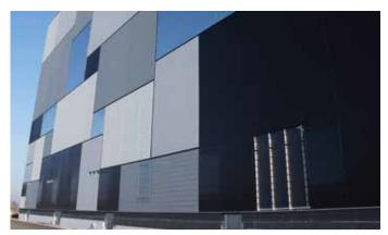
Direction-depending installation of the Kalzip FC panels...
